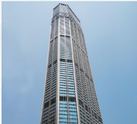
Dalian International Trade Center Building
