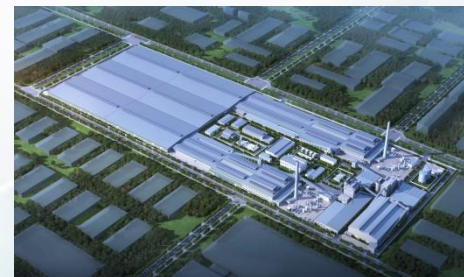
Indonesia Industrial Park (Under construction)
