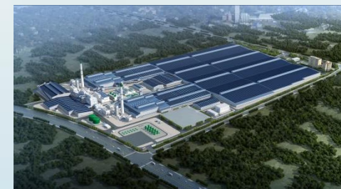
Shangrao Industrial Park (Under construction)
